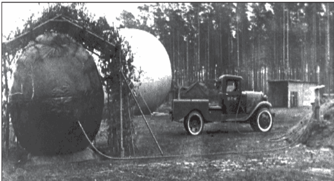
Fig. 3. Winch truck on the chassis GAS-AA on the stand. At the left – gas-holder with the “used” hydrogen, behind – the aerostat.
